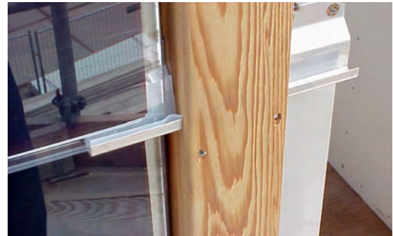
Detail of wood curtain wall and PV shingle connection under construction
