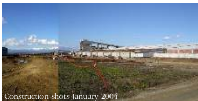
Construction shots January 2004
