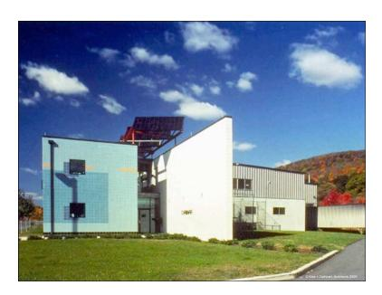
PV manufacturing facility, Port Jervis, New York 1984. Skylit hall separates office/lab area from production area; PV array prevents direct sunlight from reaching production floor.
