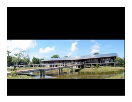
Research facility for the Smithsonian Tropical Research Institute, Bocas del Toro, Panama, 2003. Closest built project by K+C to zero-impact: produces majority of energy from PV roof, collects water for building use from the same roof, will include and onsite biological waste treatment system.
