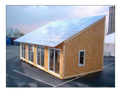
Earth day 2000 SIPS Pavilion, Battery Park City, New York, April 2000. Pavilion features a 3kW PV roof, passive solar design principles.
