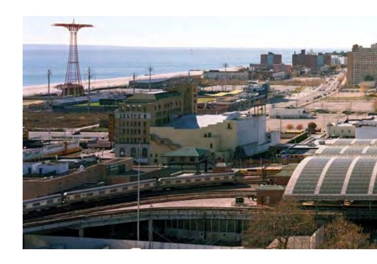
Coney Island's Stillwell Avenue Terminal is the largest above—ground station in the New York City subway system. For the reconstruction of this major intermodal terminal, Kiss + Cathcart designed a 76,000 square foot glass and steel structure using an innovative, panelized construction system of semi-transparent photovoltaic modules. These solar modules function both as enclosure and a source of approximately 200,000 kilowatt hours per year of renewable electricity.
